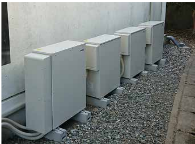
■ Figure 5: Installed storage batteries (Murata Manufacturing Co., Ltd.)
