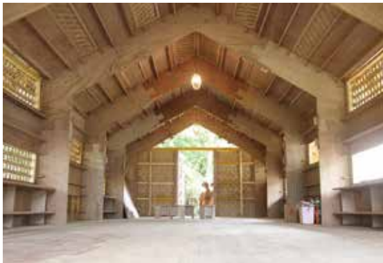
■ Photo 5: Low-cost construction of public office buildings built with digital fabrication facilities designed by Keio University
